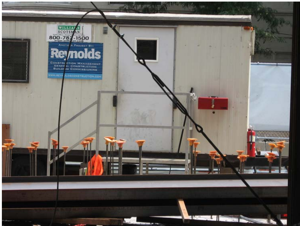
Temporary office trailer on the East corner of the project site, facing Market Street.
