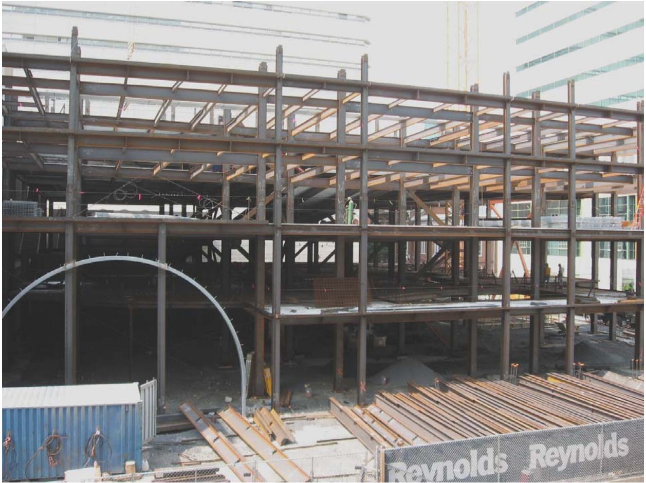
Photo taken 08.15.2007 from Market Street, South corner of site
